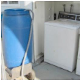
from my washing machine. I can either hook it into the existing drain on the wall, or I can hook it over the edge of a 50-gallon barrel which is on a wheeled cart. The cart can
